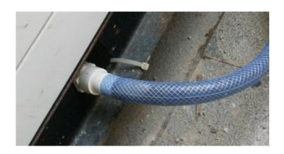
Water outlet is used for condensed water coming out of the air conditioner unit.
